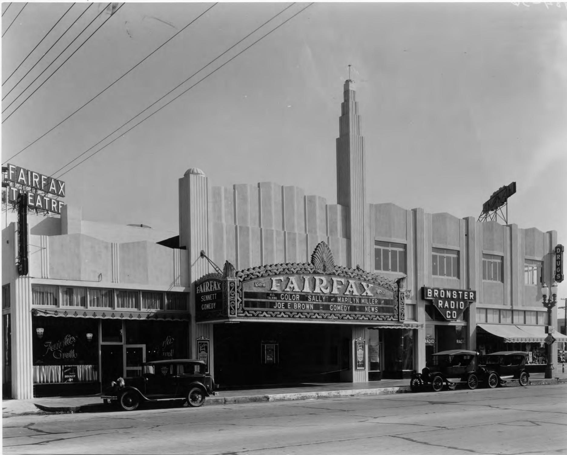
Fairfax Theatre, north view. (Mott Studios 1932)
