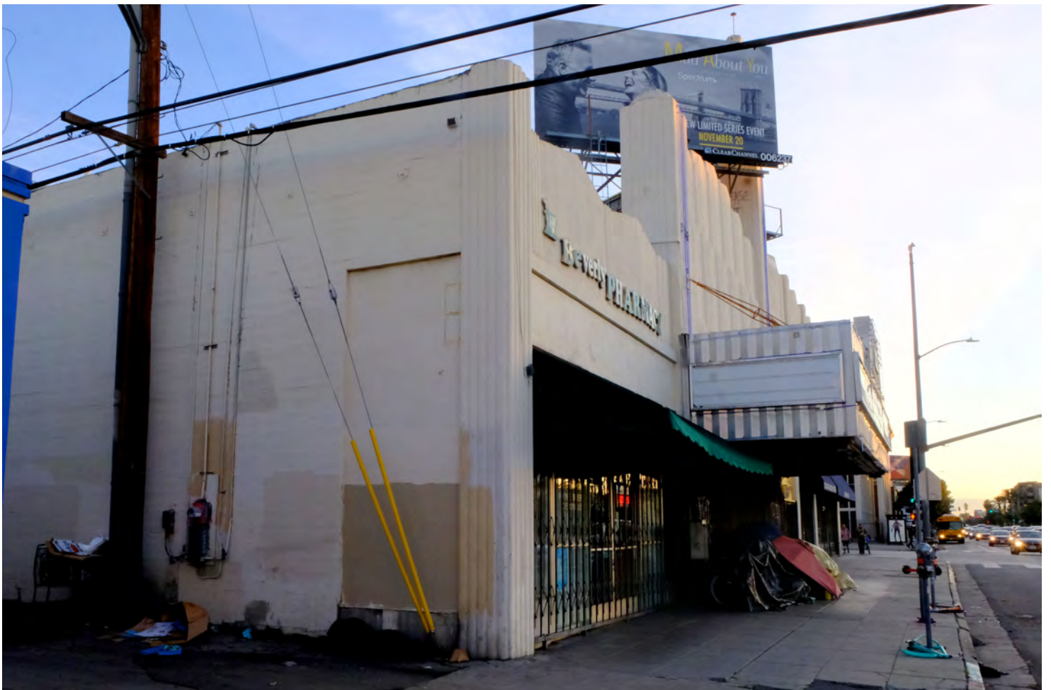
South and west façades. View east. (Luftman 2019)
