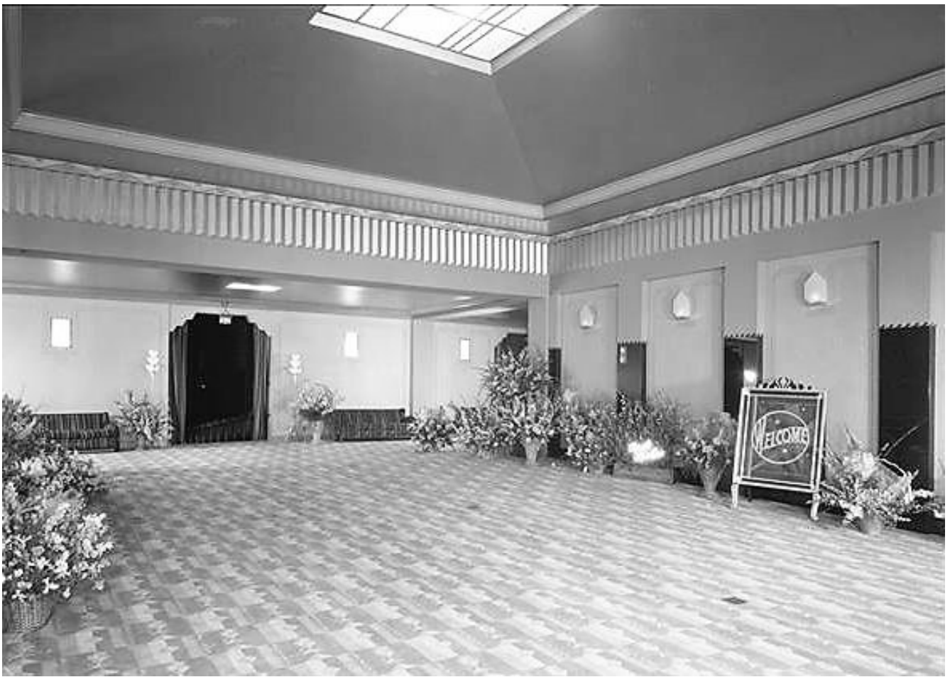
Lobby, northeast view. The Art Deco lighting fixture, dentals along the ceiling, and entryway to the auditorium were all extant when last seen. (Circa 1930)
