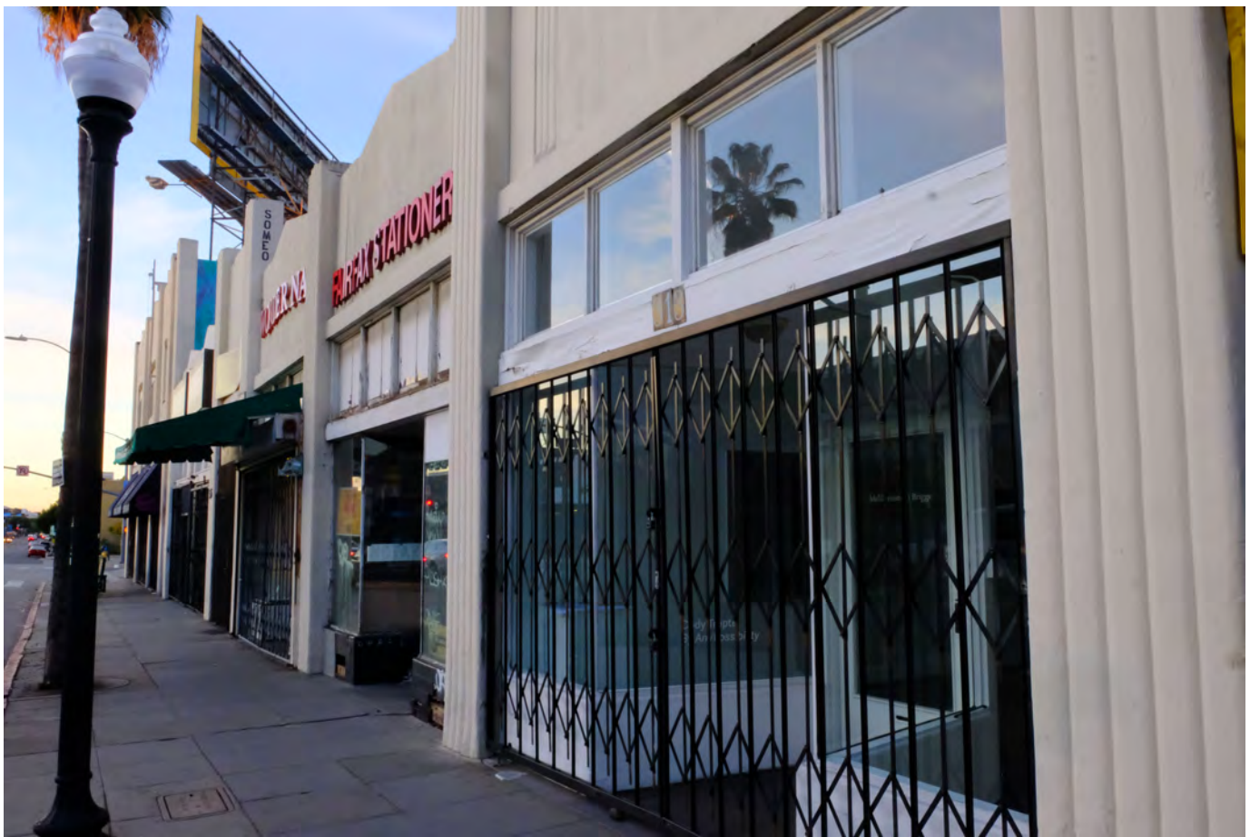
East façade, view southwest. Fluted pilasters divide the façade into storefront bays. Wood-framed hopper opening transom windows are original to the building. (Luftman 2019)
