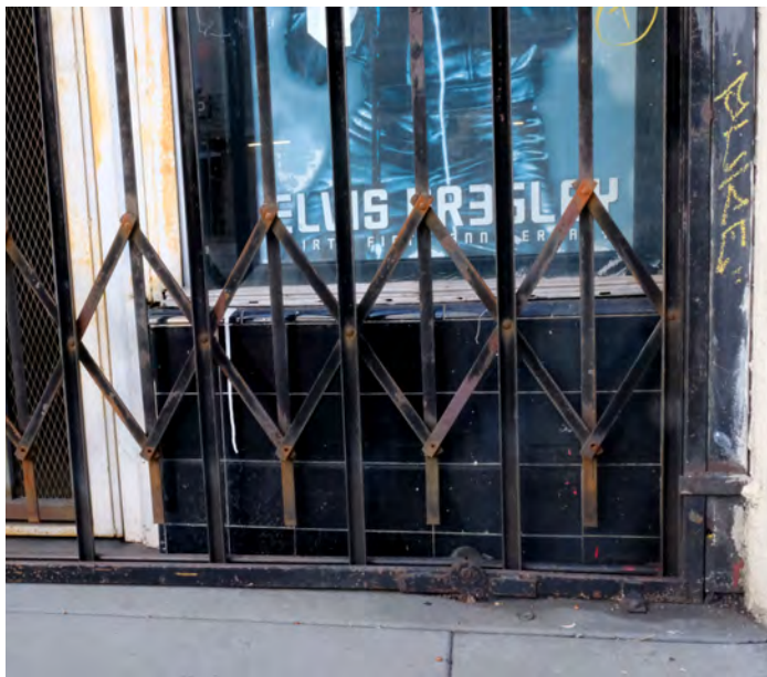
The black tiles at the base of the storefront windows are original to the building. (Luftman 2019)
